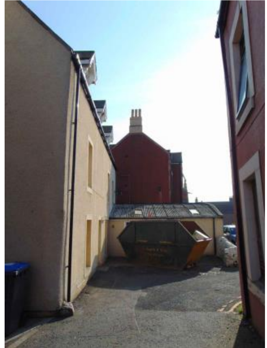
Figure 4: Image of Existing Site (western façade of the property)
