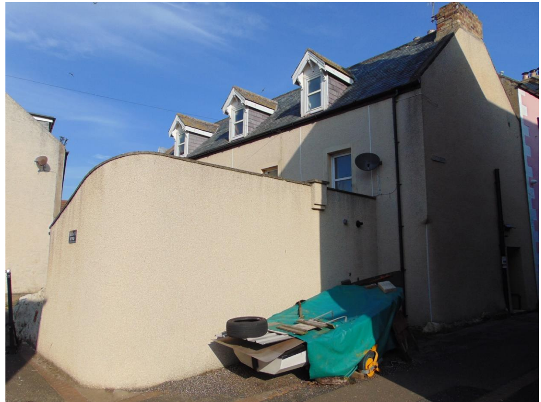
Figure 6: Image of Existing Site (eastern façade)
